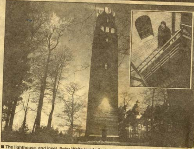
■ The lighthouse, and inset, Peter White inside the building
